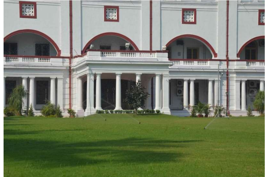
Sprinkler System in Lawn
